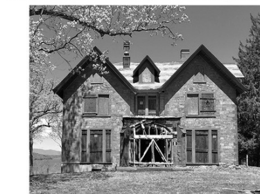
The Point after view-clearing
