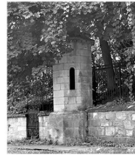
A remaining gate and wall at Highland Gardens
