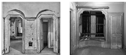
Canted corners on the doorways and a window seat on the second floor of The Point
